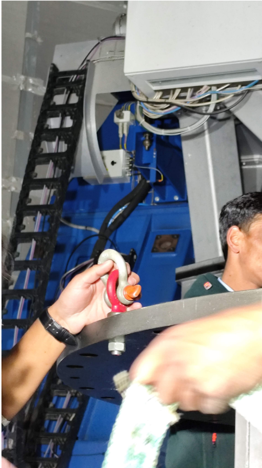
Figure 20: Attach the hooks to the instrument for its connection with the crane pulley.
