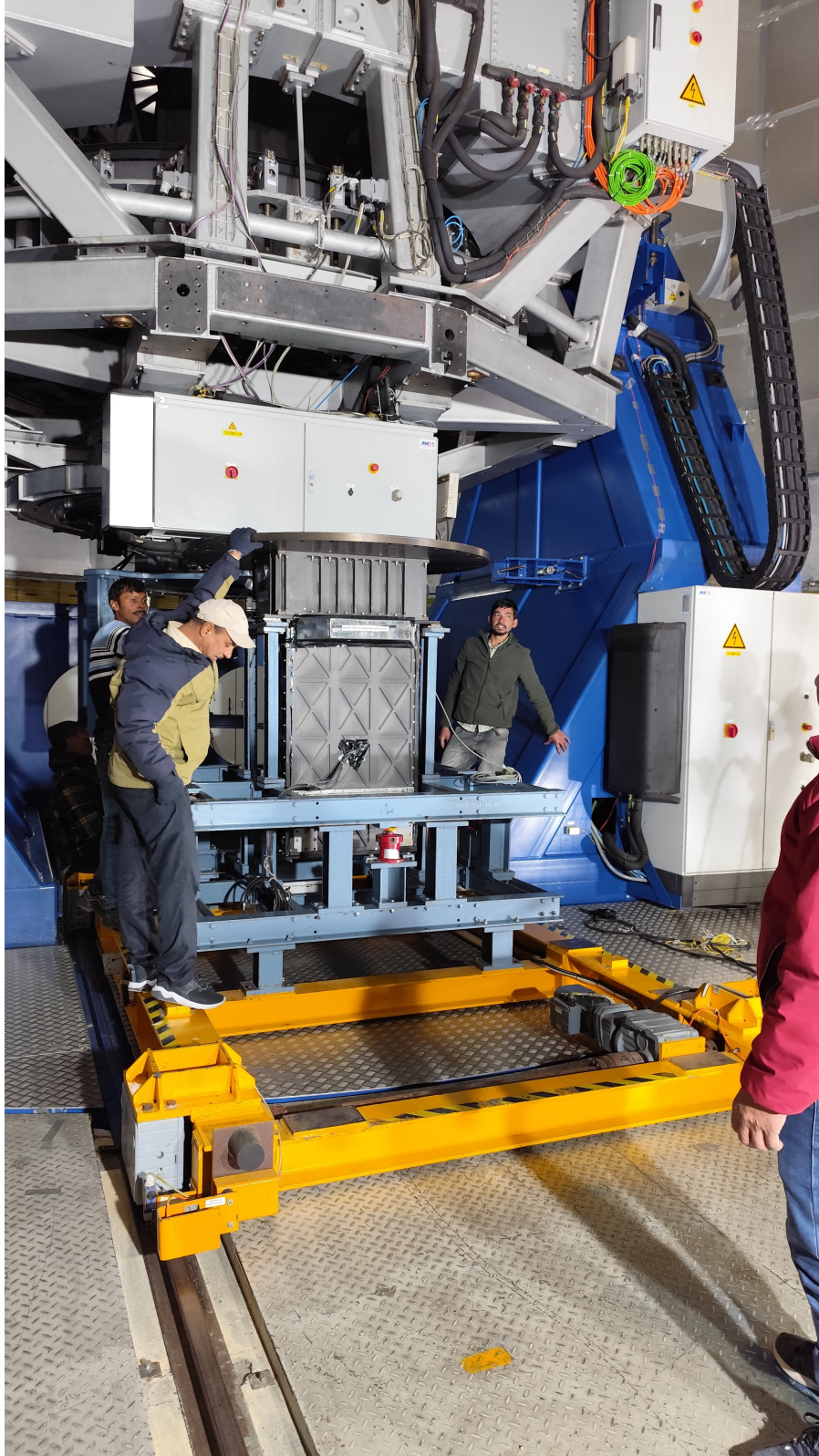
Figure 18: Move the transfer trolley holding the instrument backwards.
