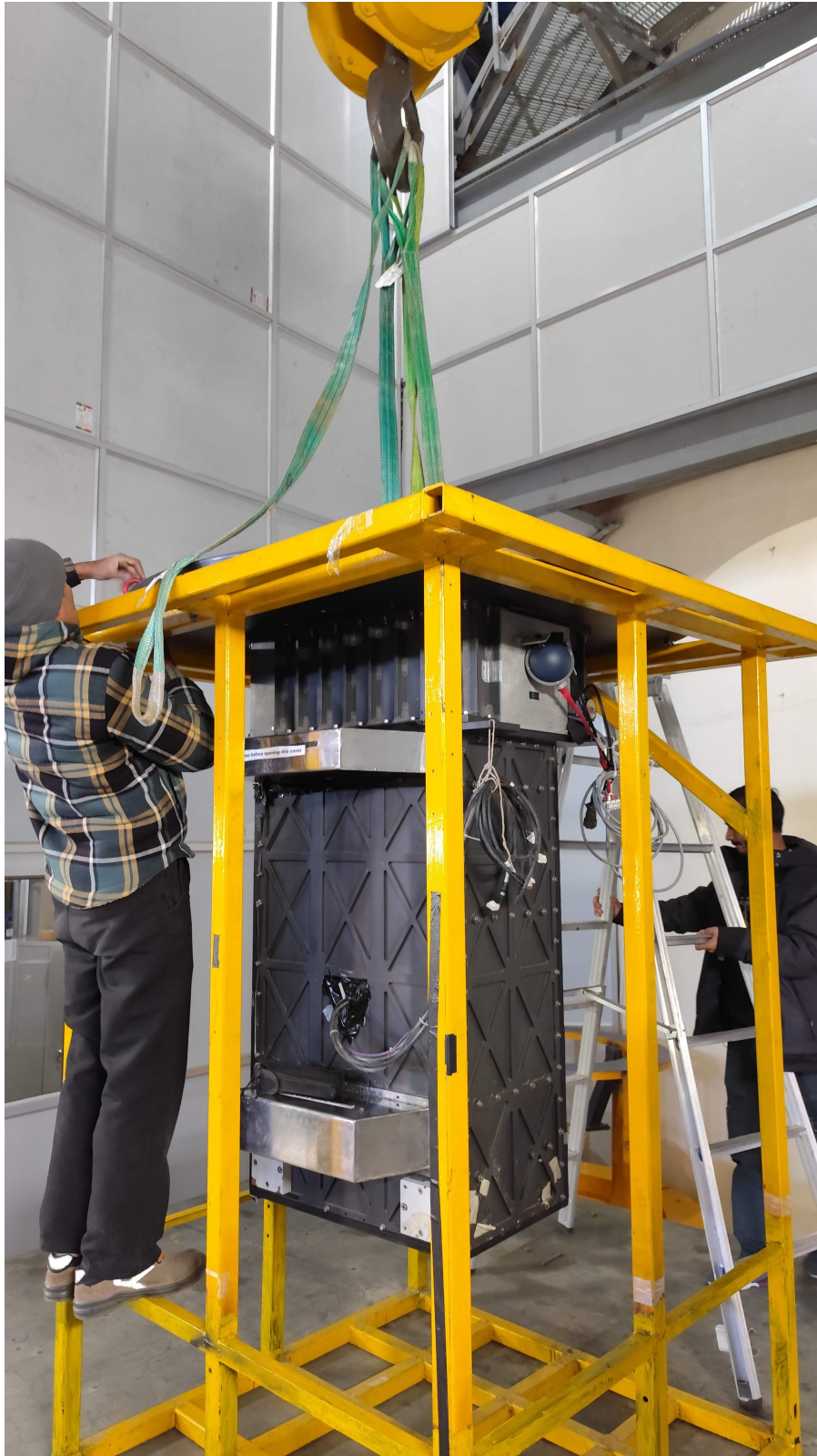
Figure 23: Remove the slings and hooks from the instrument.
