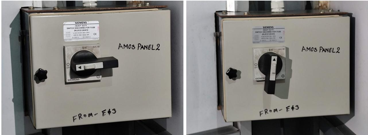
Figure 1: The OFF and ON positions of the knob in AMOS-Panel-2.
