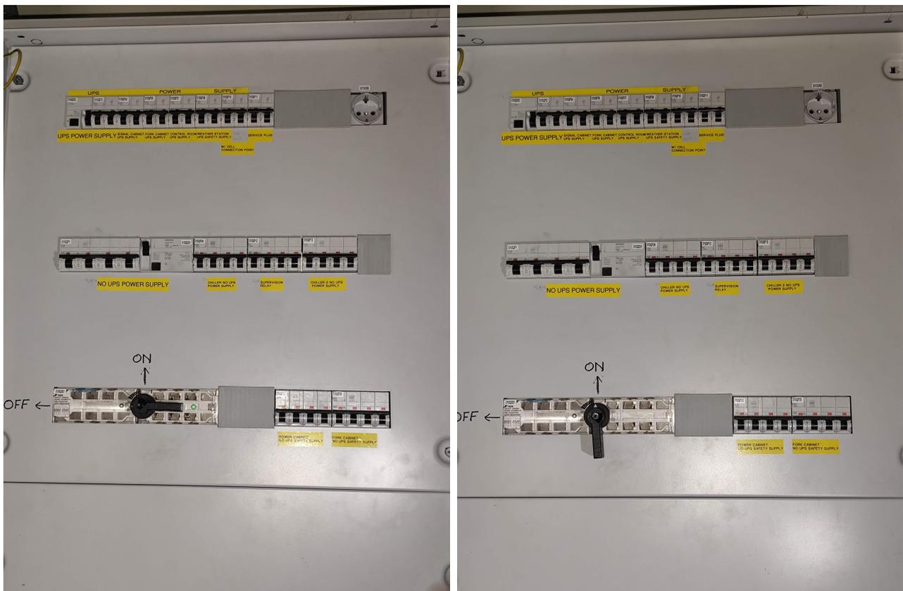
Figure 3: The OFF and ON positions of the knob in the power supply panel.
