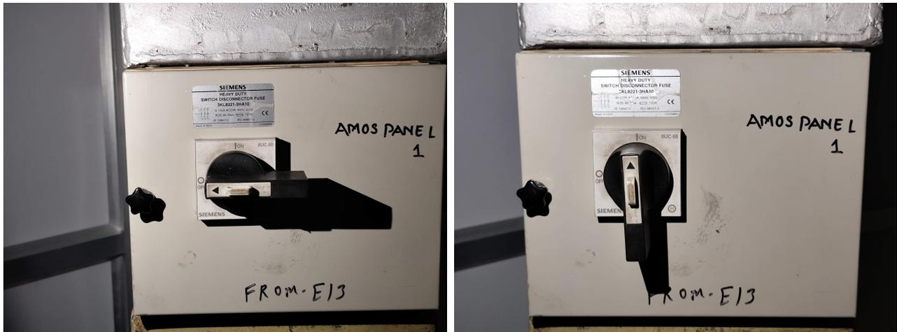
Figure 2: The OFF and ON positions of the knob in AMOS-Panel-1.
