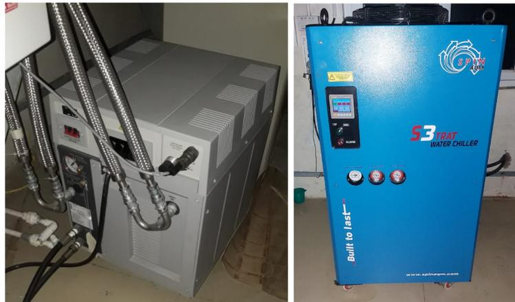
**Figure 4:** Image of Brooks high voltage model 9600 Compressor (left) and the distilled water-based Chiller (right).
