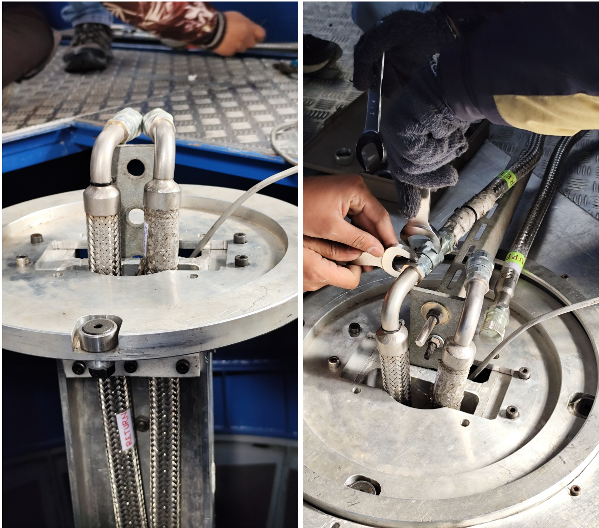
Figure 8: The compressor supply and return pipes coming from the port below the telescope. The supply and return pipes of the coolant are connected to the compressor.
