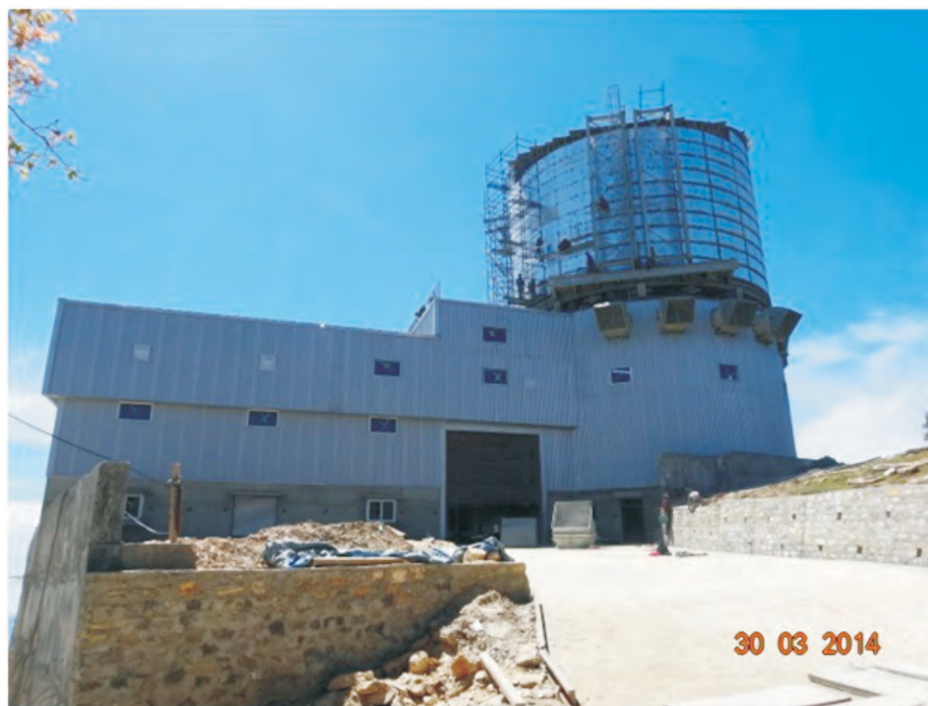
Figure 41. Picture of 3.6m building taken on 30 th March 2014. Dome support and extension building is completed. Dome structure is nearly complete.
