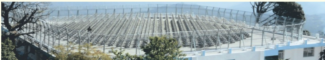
Figure 40. Recently installed clutter fence along the periphery of ASTRAD antenna array on the roof-top of the ASTRAD building.
