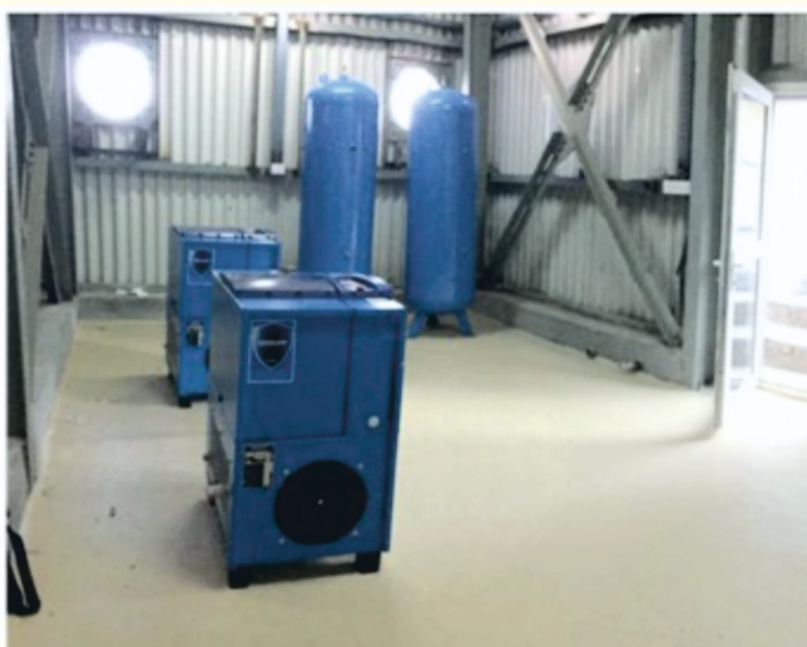
Figure 34. Compressor room with the two air compressors and air tanks.
