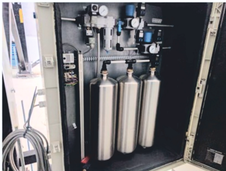
Figure 36. The AMOS pneumatic air control system installed in the ILMT control room.
