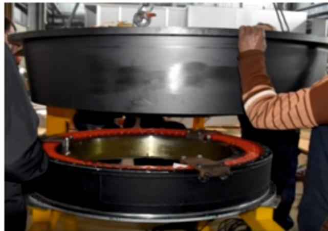
**Figure 66.** Alignment of new motor in GIS for replacement.
