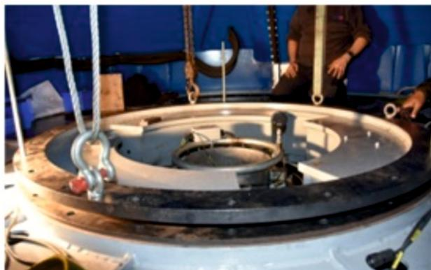
**Figure 65.** Taking out old motor.
