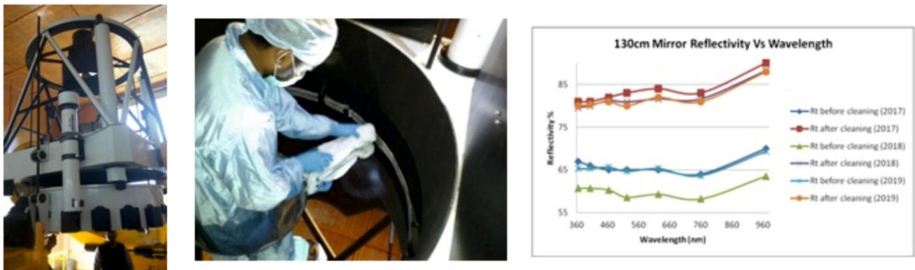
**Figure 62.** 1.3m telescope M1 cell un-mounting (left), Cleaning process (middle), M1 Reflectivity (right).
