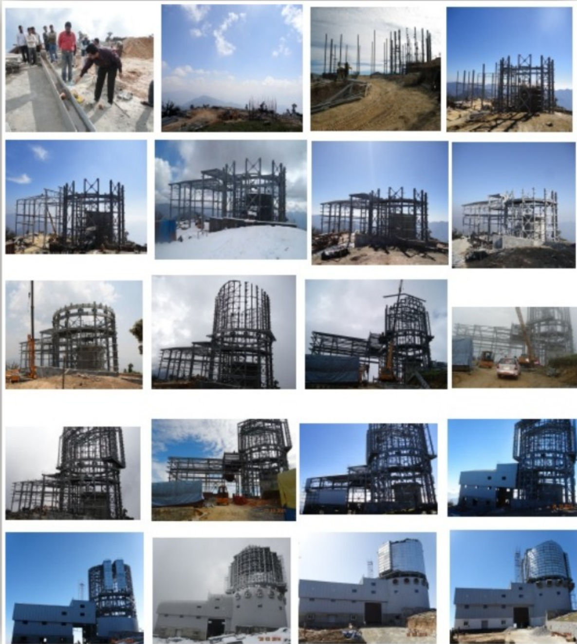
Figure 36. Timeline of telescope enclosure building construction. Month 1 to month 20 row wise. The erection of building was completed in 22 months.
