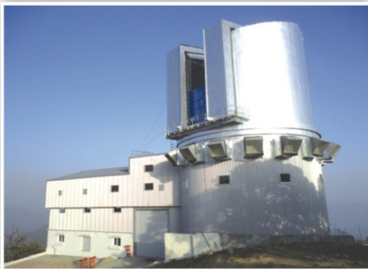
Figure 34: Picture of as-built 3.6m Telescope Enclosure building taken in July 2014. The dome has been completed during the financial year. The dome slit is open and the wind-screen (blue) can be seen.
