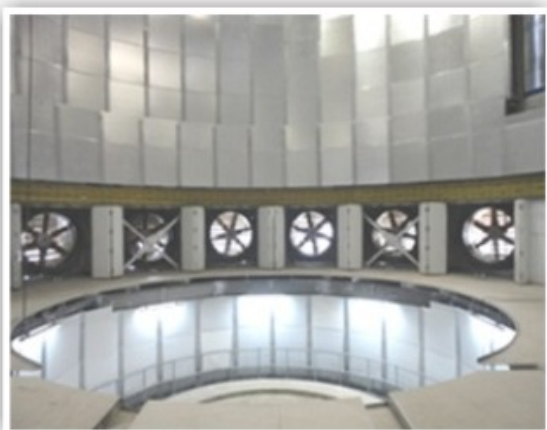
Figure 62. View of the vents from inside the dome housing before the telescope was installed.
