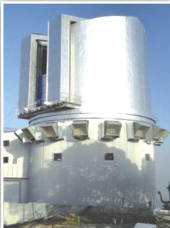
Figure 60. The cylindrical dome structure with tapering roof. The slit of the dome is kept open. Fan operated vents are seen on the dome structure. View of these vents from inside the dome is shown below.
