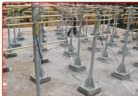
**Figure 32.** Work is in progress for the mini profiler (49 subarray) at ECIL, Hyderabad.
