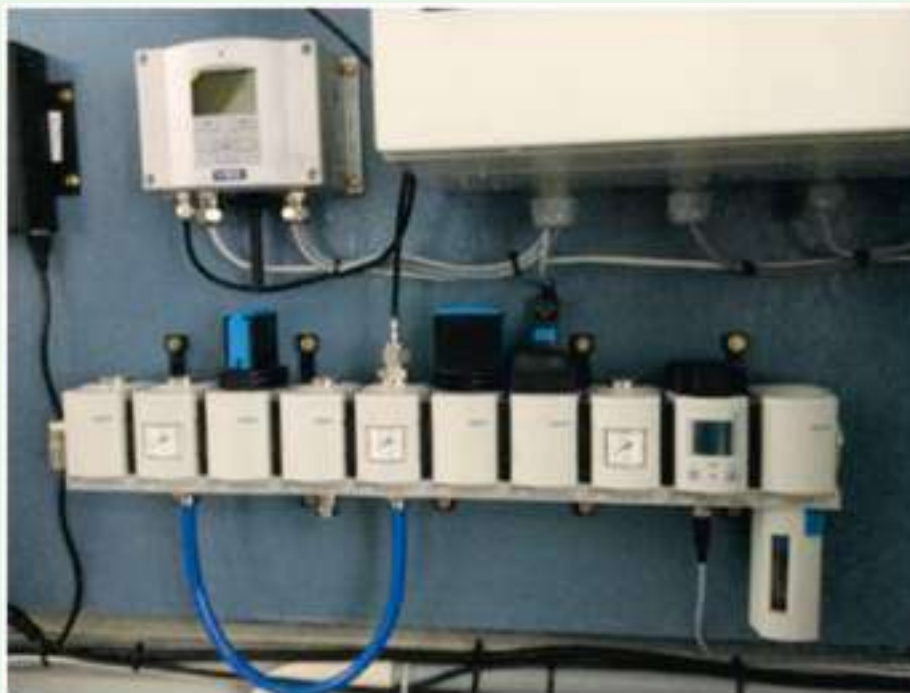
Figure 29. Filter, valve and dew point sensor installed for the control of pneumatic system.
