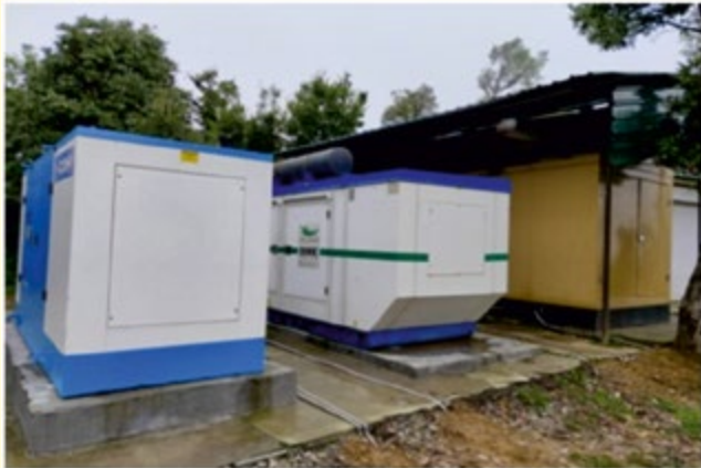
Figure 48. 400KVA, 160KVA and 82.5 KVA DG sets at Devathal.
