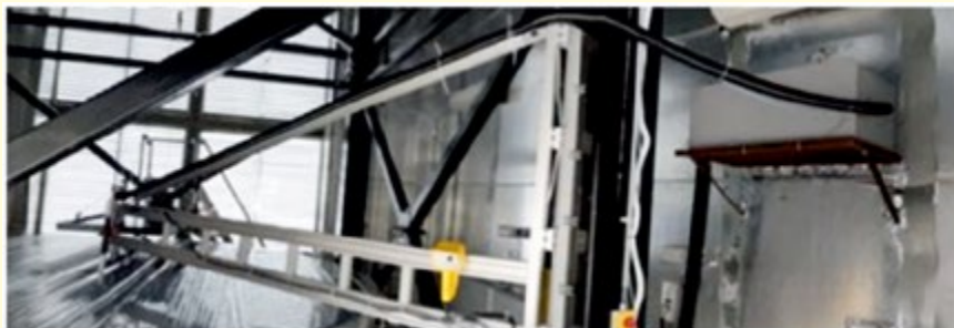
Figure 30. Hg vapour extractor located on a brown platform at right filled with carbon filter. One end of the black pipe is connected to the extractor and the other end goes near the center of the primary mirror.
