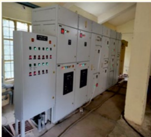
Figure 44. 400KVA SCADA based substation at Devasthal.
