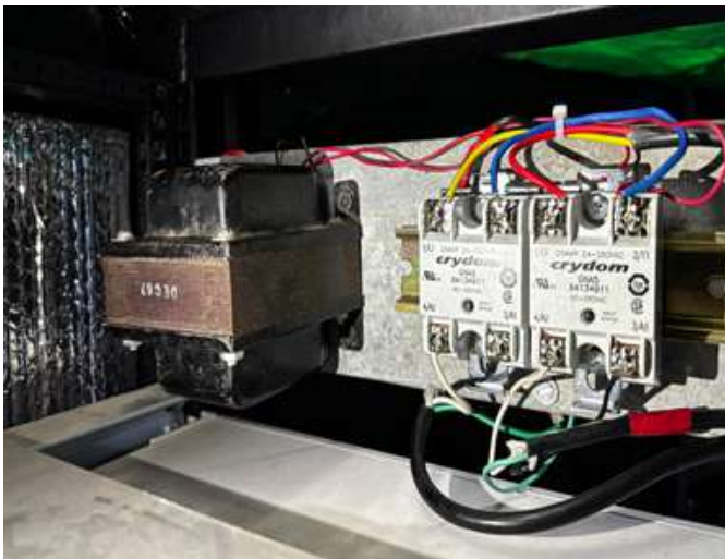
Figure 91. SSR relay mounted inside the TANSPEC instrument enclosure.
